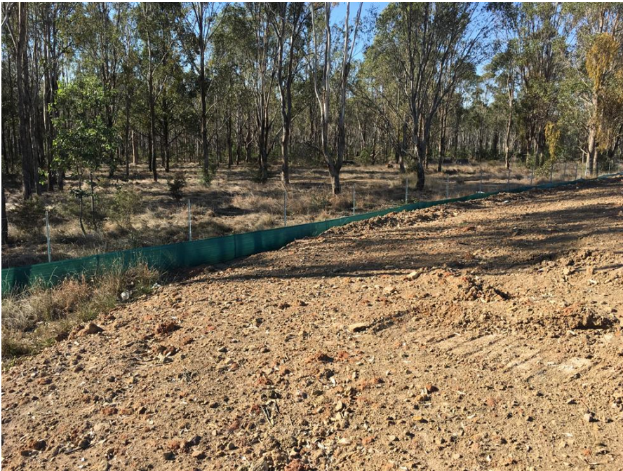
Figure 2: Phytophthora cinnamomi controls along the boundary of the BioBank site
