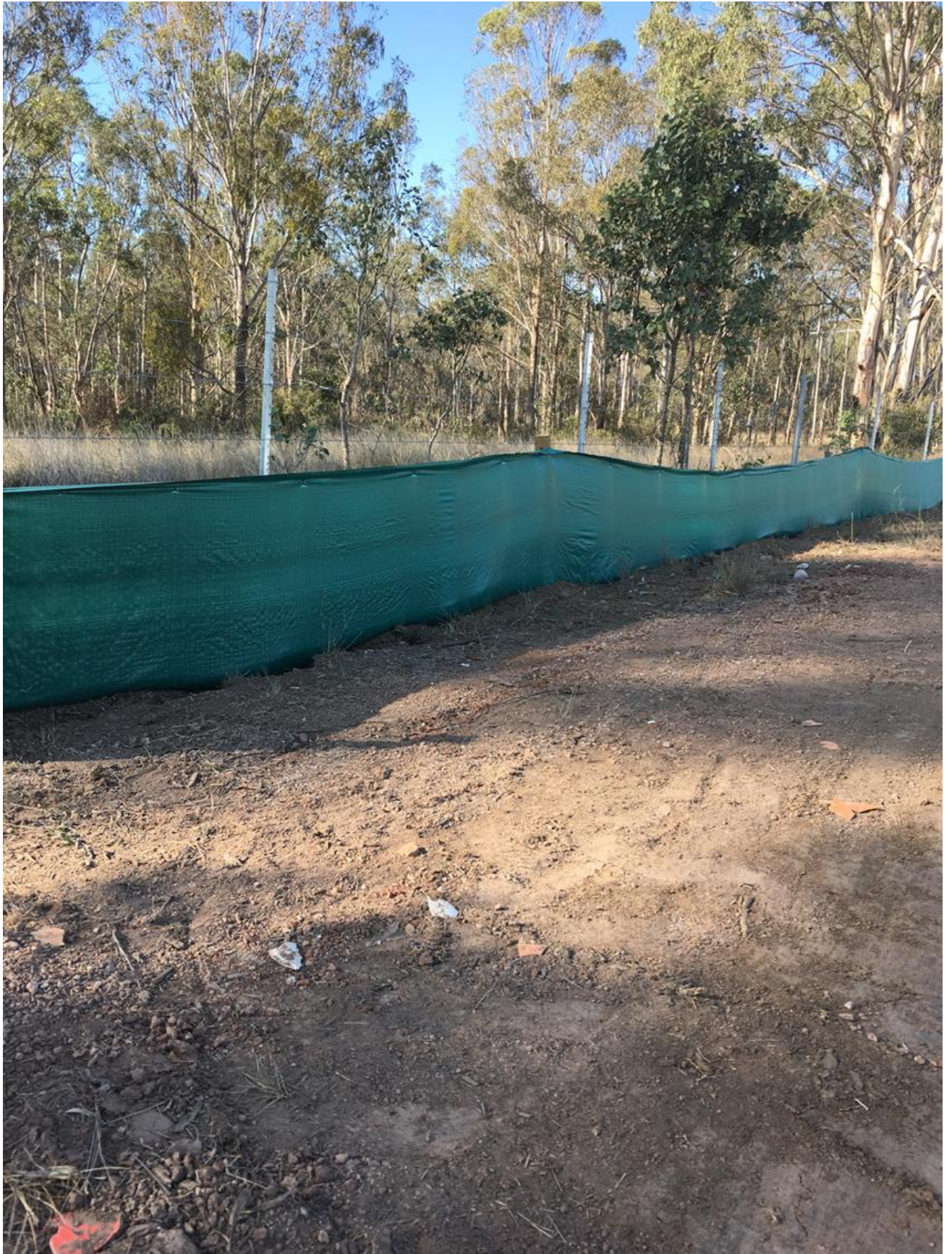
Figure 3: Phytophthora cinnamomi controls preventing runoff from the development footprint into the BioBank Site
