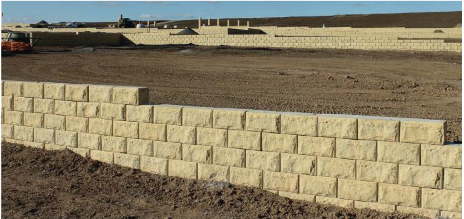
Photo of Retaining Walls in Emerald Hills Constructed by Macarthur Developments
